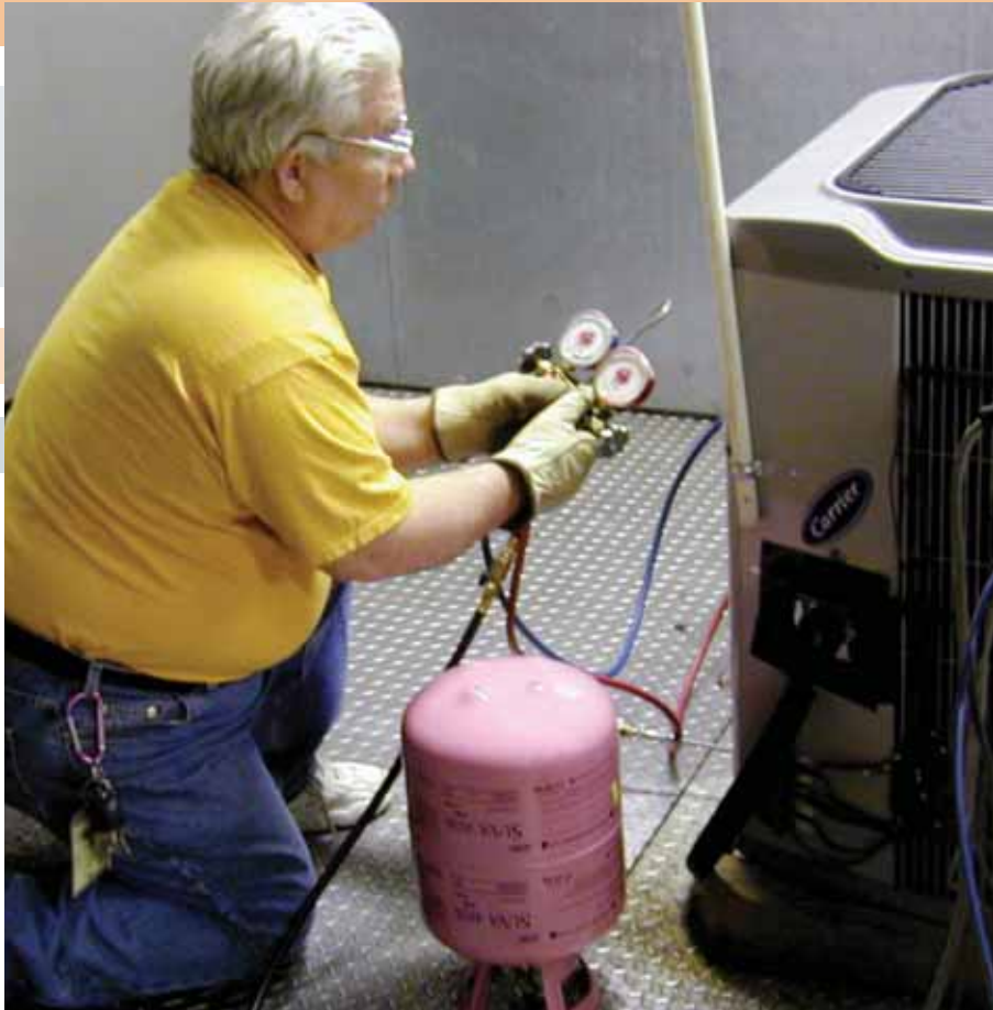
Working with R-410A is not much different than any other refrigerant. However, R-410A does have higher pressure and can become combustible when mixed with air.
